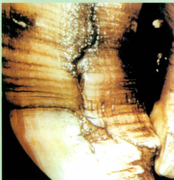
Figura 8. Rachadura vertical. (GREENOUGH e WEAVER, 1997).
